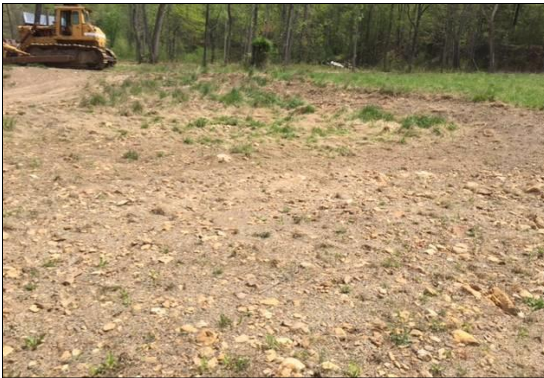
Figure 7-37: Access road in area of ponds near Tredegar House.
