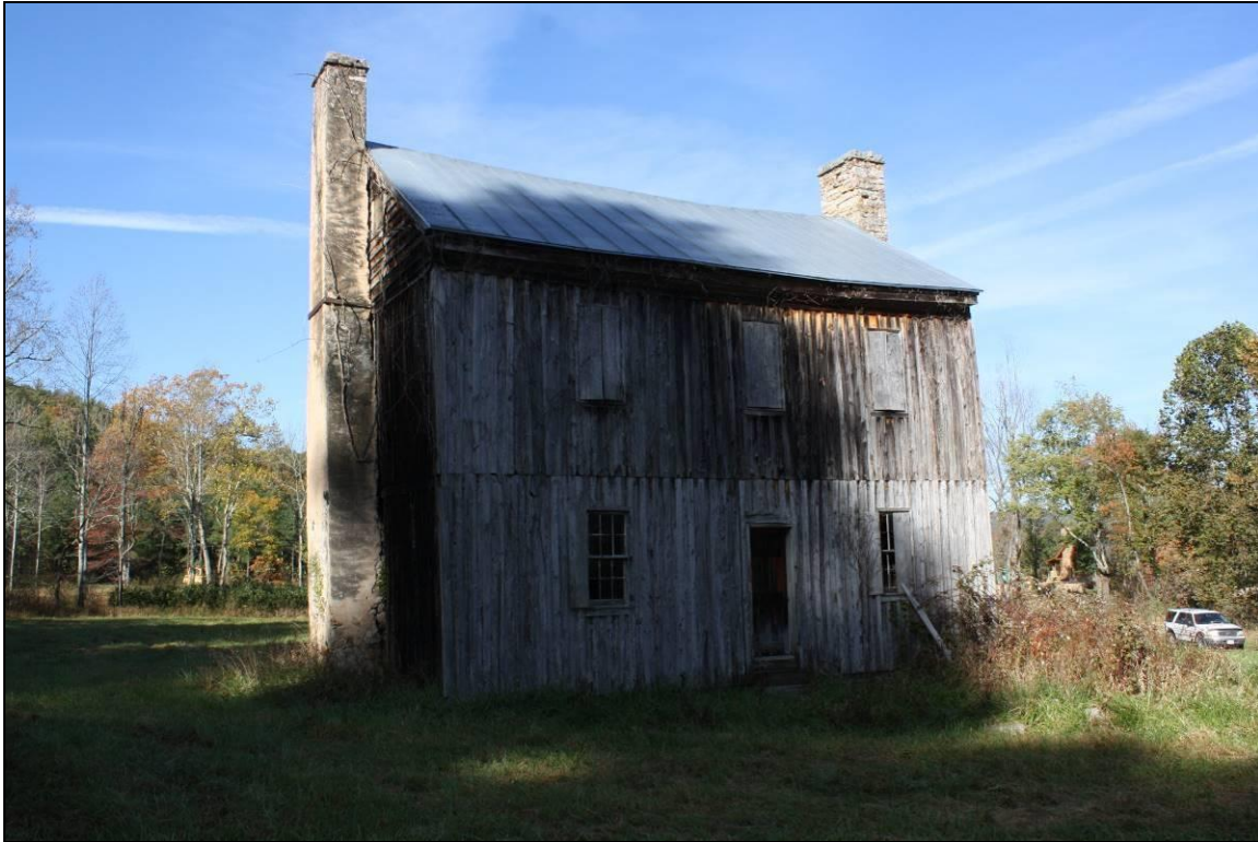
Figure 7-5: Tredegar House, east façade, facing northwest
