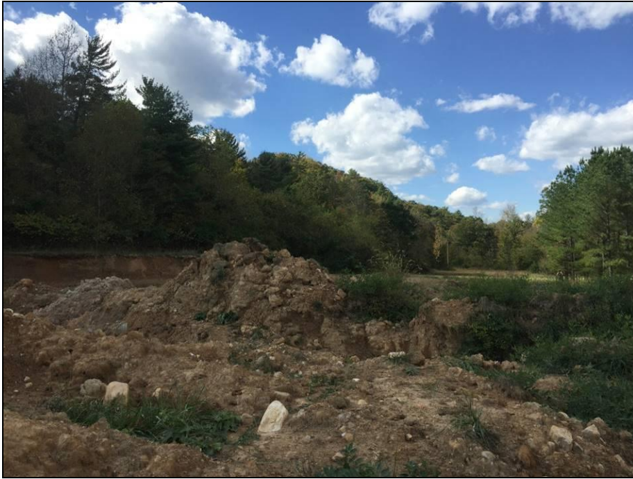
Figure 7-18: Graded area in Laydown Yard/O&M 1, looking west.
