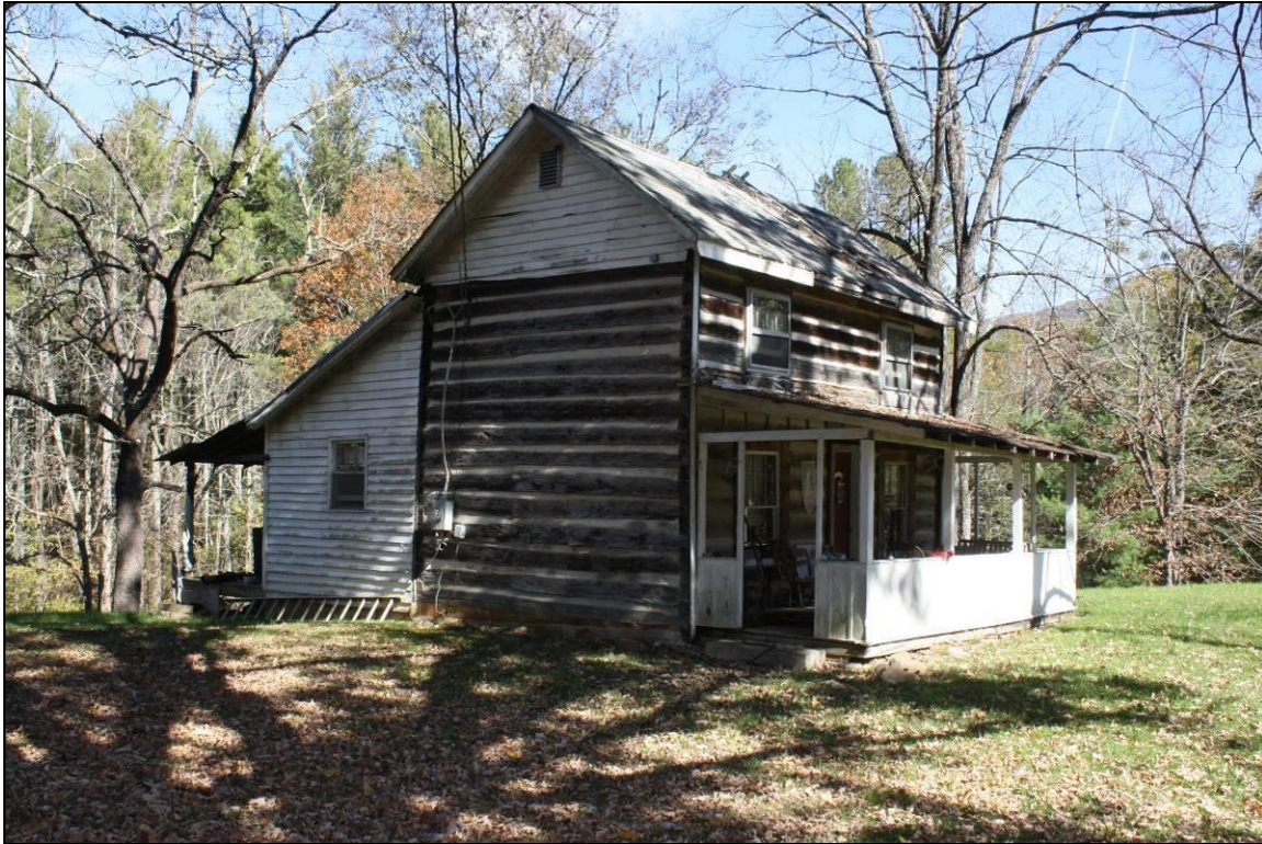
Figure 7-14: 2905 Daggers Springs Road, front and west side, facing northeast
