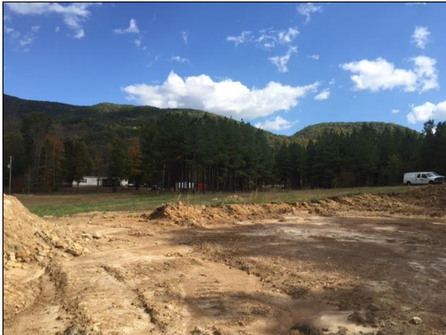
Figure 7-17: Graded area in Laydown Yard/O&M 1, looking east.
